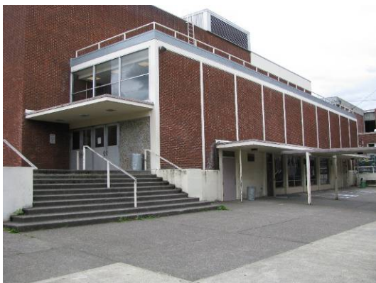
Entrance to new gymnasium (213B), looking Northeast.
