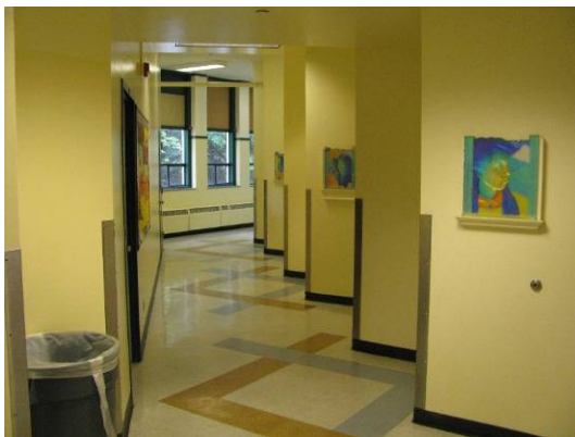
Alterations to south corridor (213A).
