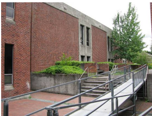
Classroom addition (213D), looking east.
