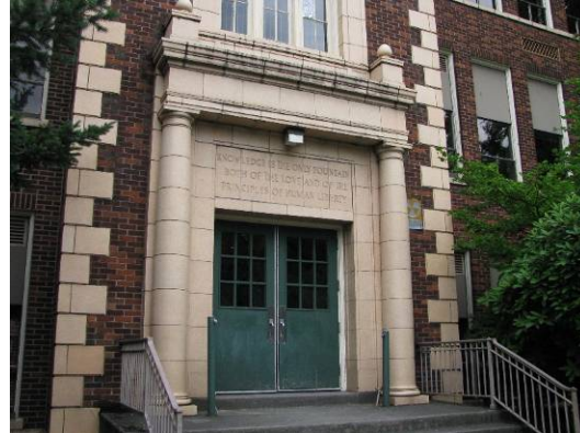
Typical side entrance, north side entrance, main school building (213A).
