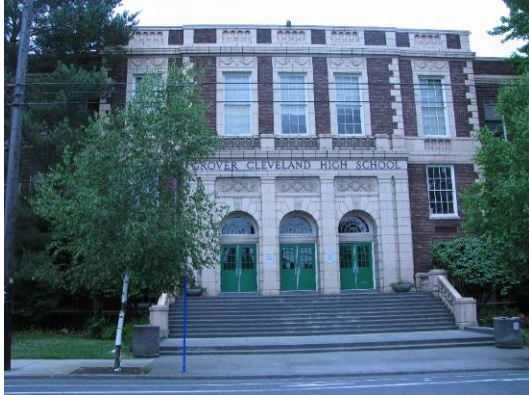
Principal (west) elevation, main entrance (213A).
